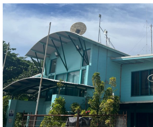
Figure 11: TSIRC building with nbn Sky Muster dish and Wi-Fi access point on roof
