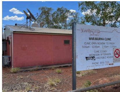
Figures 30 & 31: Warakurna Roadhouse and Warakurna Clinic
